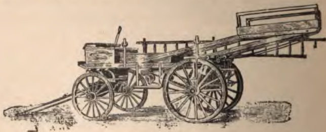
FIG. 245.—Tower wagon for use in repairing pole lines.
